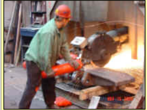
Swing Grinding the Riser Stubs
