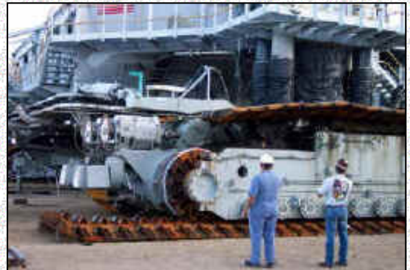
Track Belt Being Installed on the Transporter
