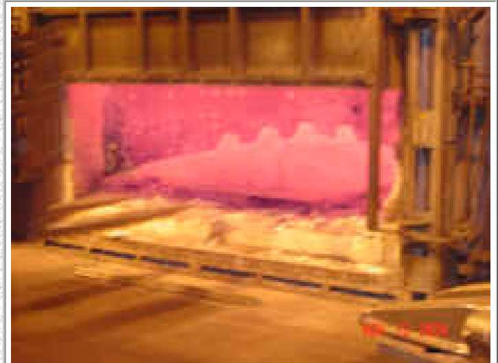
Pacific Steel Heat Treat Furnace
